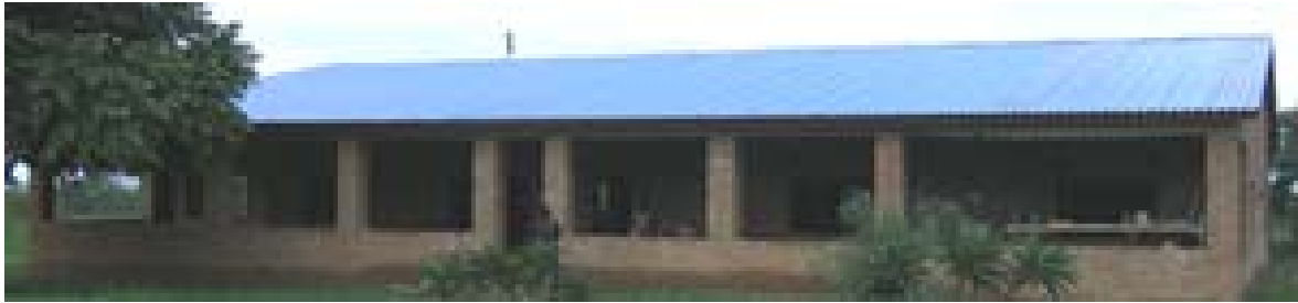
Kelly's House with unfinished walls and roof
